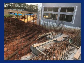
Retaining wall footers and reinforcement at lower level entrance
