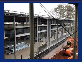
2<sup>nd</sup> level east exterior framing in progress (south elevation)
