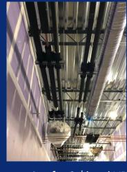
Line sets starting for 3<sup>rd</sup> level VRF system
